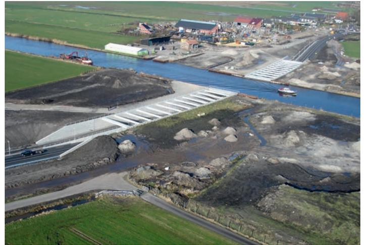
Figure 8. Aerial view of the Frisian Lakes Project: The new roadway goes under the canal which improves traffic flow.
